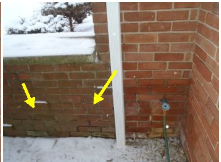
Front Door: Cracking at brick mortar joints. Recommend repairing and tuck pointing mortar joints as needed.
