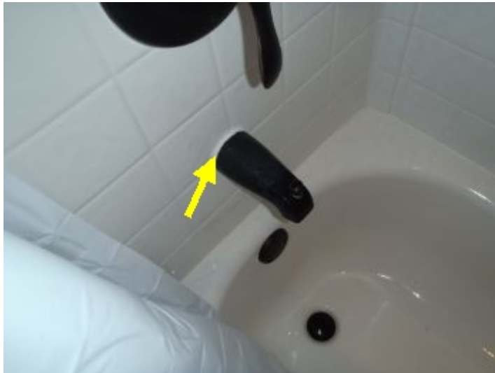
Tub spout is loose in bath 1, recommend repair as needed.
