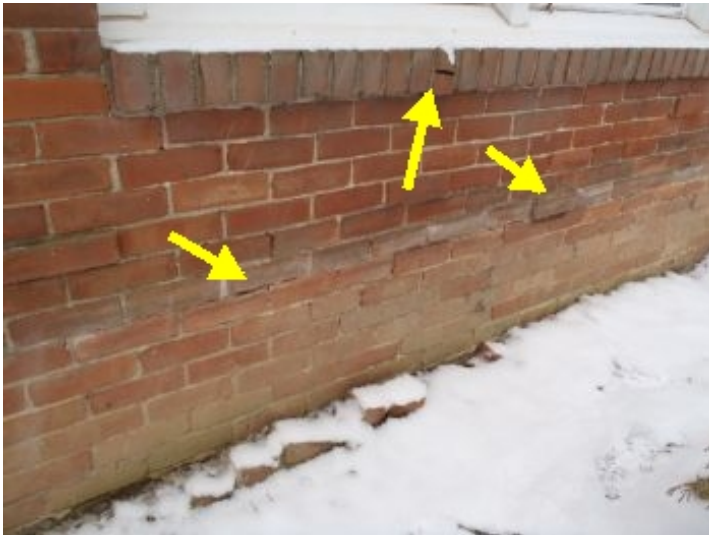
SE: Cracking at brick mortar joints. Recommend repairing and tuck pointing mortar joints as needed.
