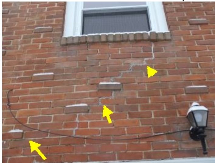
Cracking at brick mortar joints. Recommend repairing and tuck pointing mortar joints as needed.
