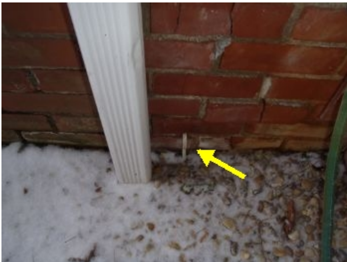
The wiring located nest to front door is susceptible to damage. It is recommended a licensed electrician review for proper installation.
