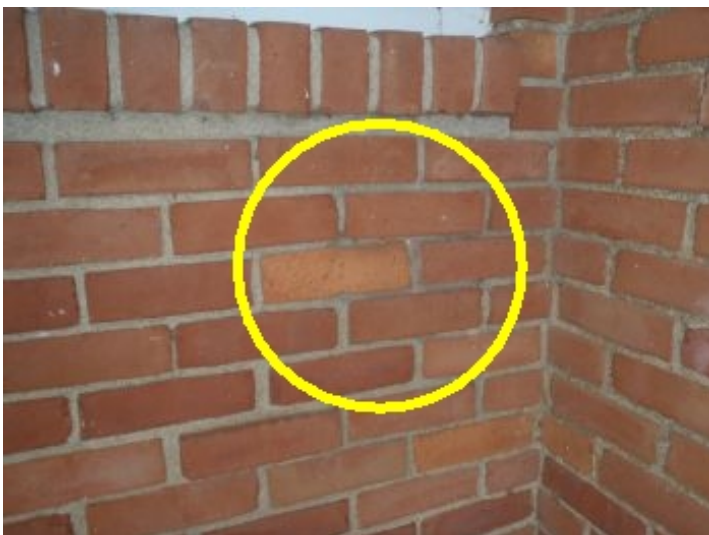
NE: Cracking at brick mortar joints. Recommend repairing and tuck pointing mortar joints as needed.
