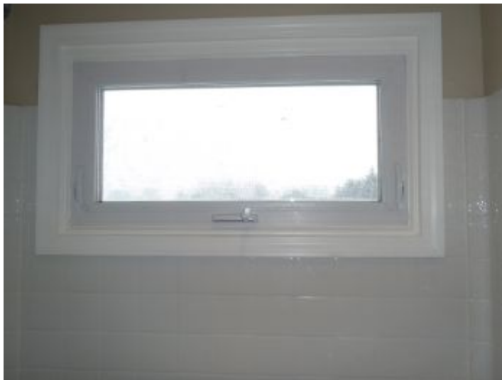
Recommend protecting shower window from water.
