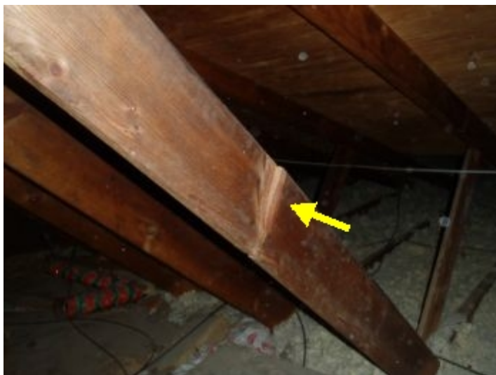
Just inside attic hole: Cracked truss brace, repair as needed.
