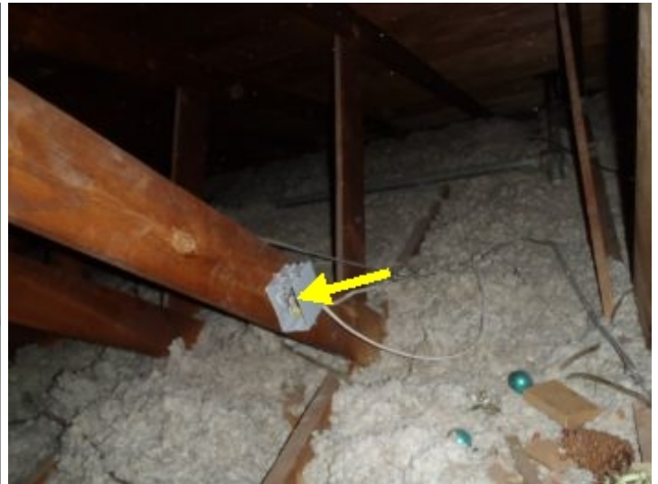
Missing junction box cover in attic. Repair as needed.
