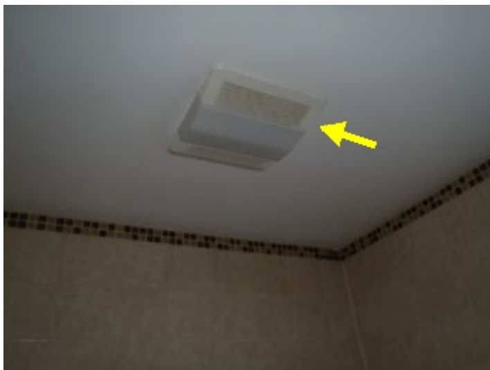
Bath 2: fan is loud, repair as needed.
