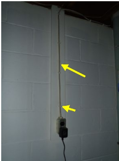
The wiring located in the basement and garage is susceptible to damage. It is recommended a licensed electrician review for proper installation.
